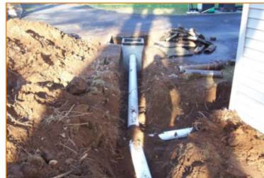
Underground Drainage System
